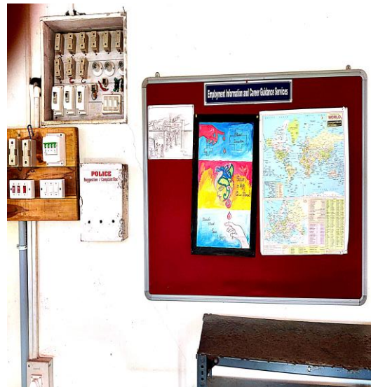
Library notice board and Complaint box
